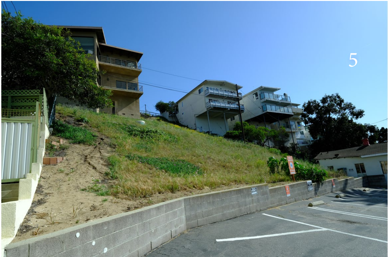
Looking south from the northeast corner of the lot
