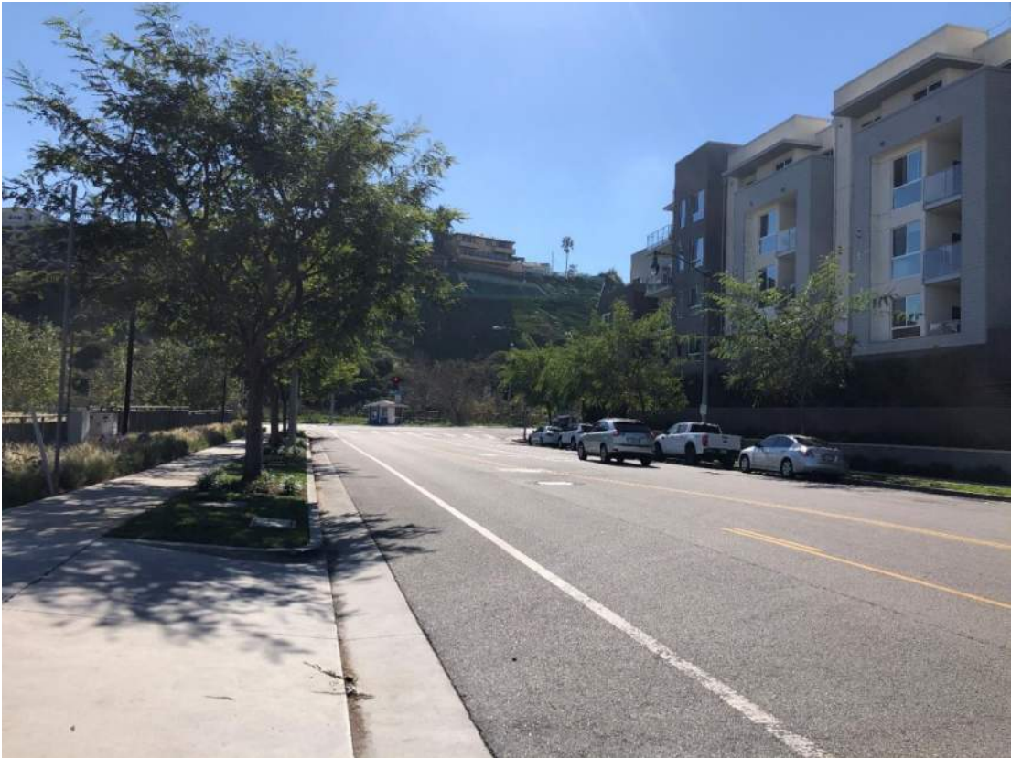
Photo 14. Southeasterly view of the public right-of-way on Westlawn Avenue and the nearby residential uses.
